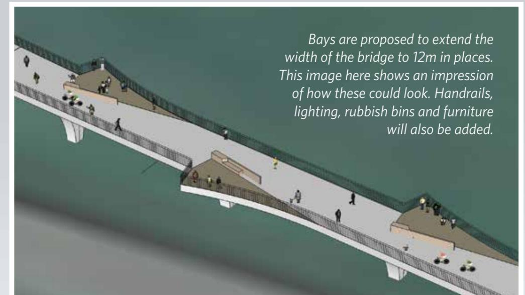
Bays are proposed to extend the width of the bridge to 12m in places. This image here shows an impression of how these could look. Handrails, lighting, rubbish bins and furniture will also be added.
